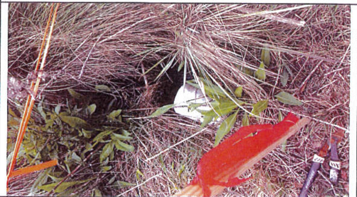
Photo 8: Drainage outfall – west side.
