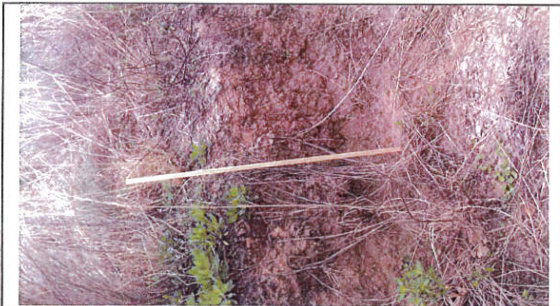
Photo 5: Slope toe erosion.
