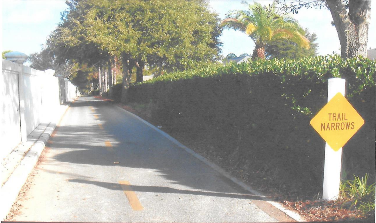
EXHIBIT 1-1 Narrow 'Feeder' Golf Cart Trail To Tunnel B4
